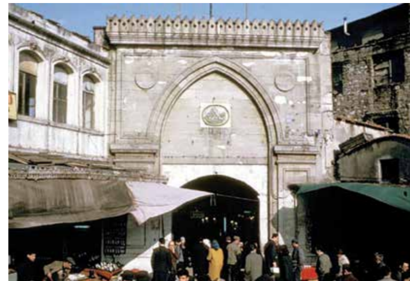
Covered Bazaar in Istanbul. View from the Beyazit Gate, leading into the Kalpakçilar Street at its western end. Above the entrance is the royal monogram (tugra) of Abdülhamid II (1876-1909), marking the construction of the gate during the 1892-94 restoration. A short Arabic phrase included in the monogram medallion says: "God loves the one who does trade".
